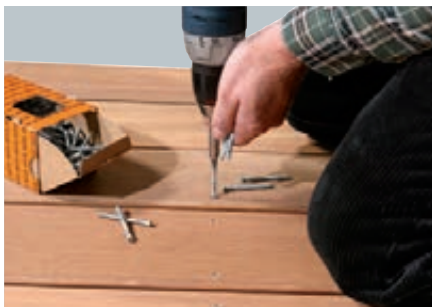
Fixing of decking
